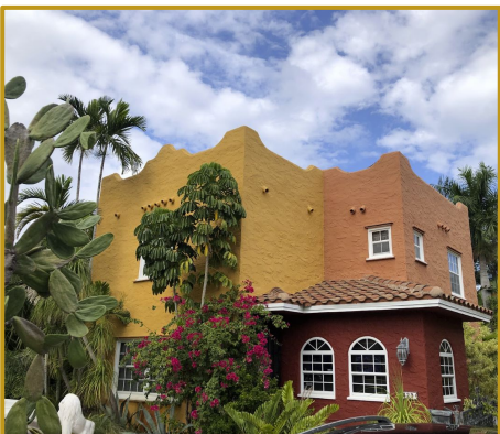
Hurricane Damage - West Palm Beach
