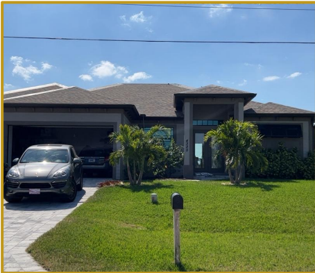
Hurricane Damage - Cape Coral
