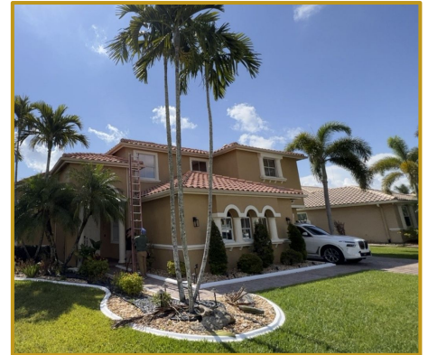
Water Damage - Pembroke Pines
